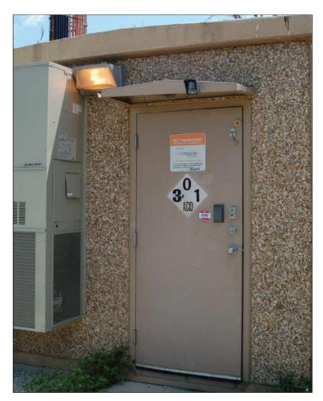
This view of a shelter shows the camera above the door and a proximity card reader on the door above the doorknob. The camera also views any approach to the air conditioner. Some thieves have removed air conditioners to gain entry to the building and have stolen all or part of the air conditioners for the metal they contain.
